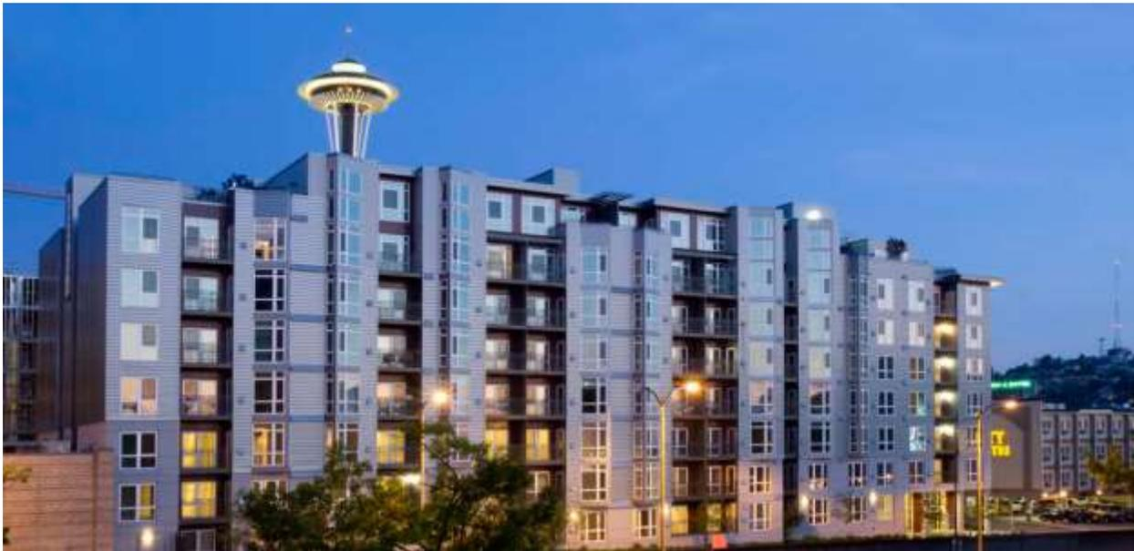
*Marselle’s 132-unit condominium building, a wood (primarily EWP) and concrete structure in Seattle. The developer reported that building the top five stories with wood saved 30% in construction costs. Photo: Matt Todd, courtesy WoodWorks.*
