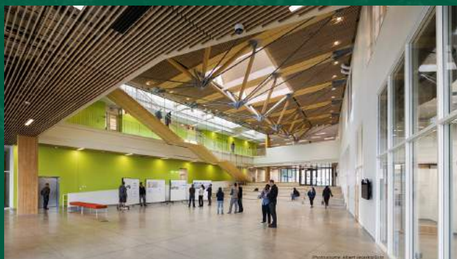
The 17-time award winning Olver Design Building at UMass - Amherst highlights the structural utility and aesthetic beauty of wood. Image courtesy of Albert Vecerka/Esto.
