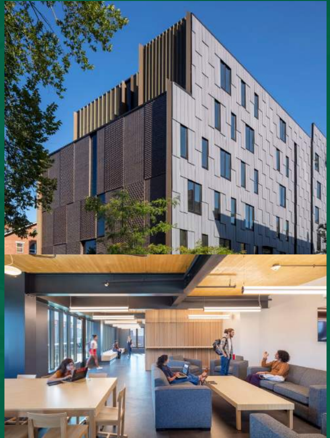
Rhode Island School of Design's North Hall, opened in 2019 with a cross-laminated timber (CLT) and steel-frame hybrid structure. Images courtesy of John Horner and NADAAA.
