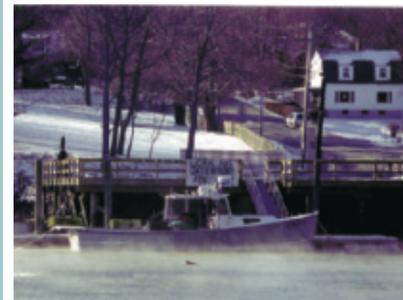
Protecting Sewall's Bridge Dock allowed the continuation of commercial fishing, important to York as a community.
