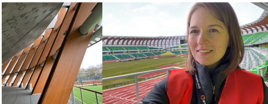
Jen toured the University of Oregon's Hayward Field to see its beautiful glulam elements made from Doug Fir. Glulam is a type of mass timber.
